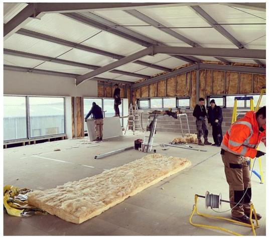
The second image shows the internal false ceiling being installed. There appears to be no sound insulation in the roof either:
